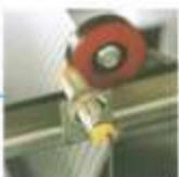
When the handrail speed versus step is slower than certain percentage, the escalator (moving walk) will be stopped for running.
